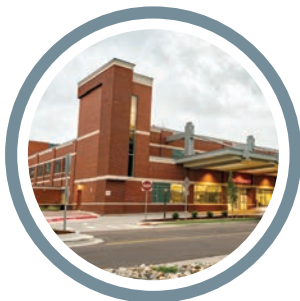
Poudre Valley Hospital 2000, 2004, 2009, 2014, 2018
